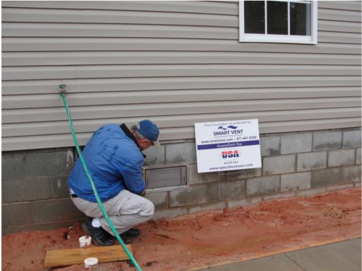
Pictured is volunteer Chip Jones installing vent.
